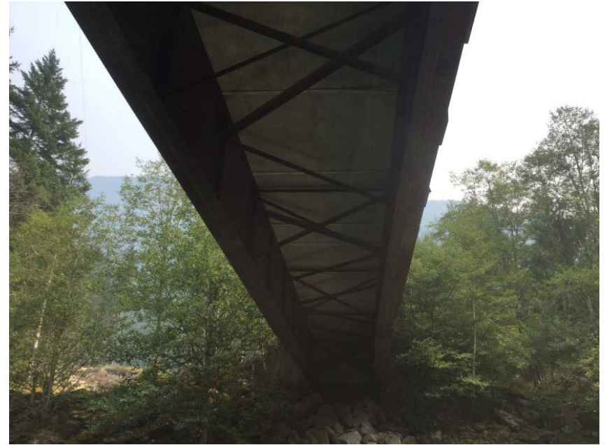
Main span superstructure
