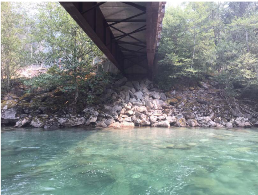
Left Bank Abutment when facing downstream
