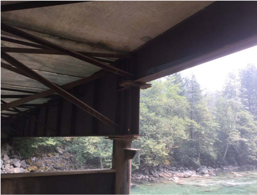
Main span to jump span connection
